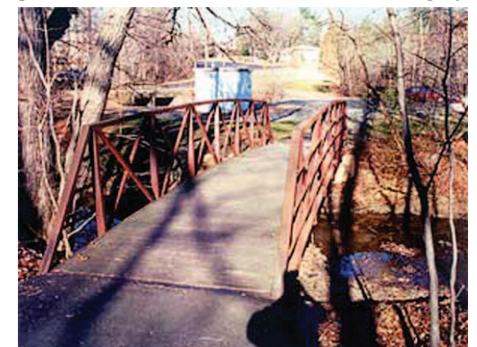
This small bridge was a drop-off point where FBI double-agent Robert Hanssen left secret documents for the KGB.
